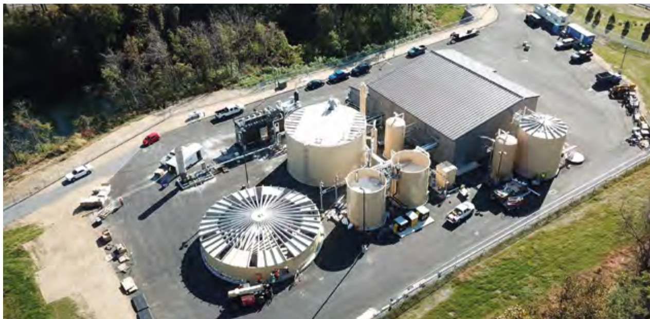
Image: New Wastewater Treatment Plant in Hershey, PA
